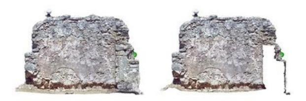
Fig.9 Understanding the irregular material loss on walls via two different sections
