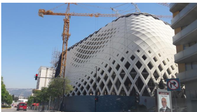
Fig. 10. Beirut Souks Mall under construction
