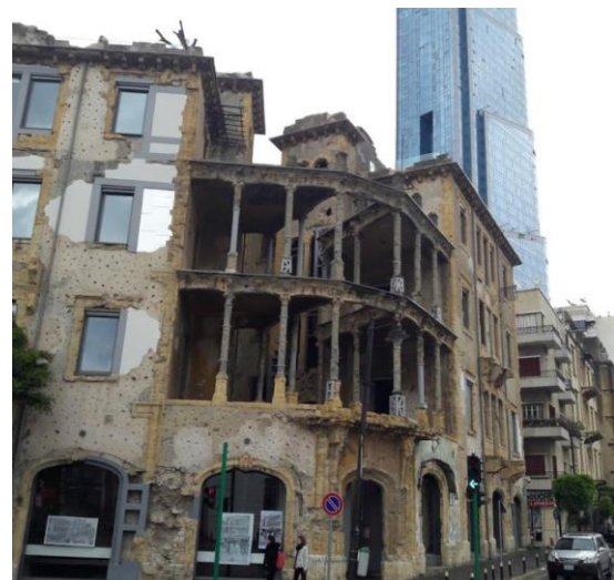
Fig. 9. Barakat Building in 2018. Now a civil war museum, the structure is one of the few buildings preserved in its war-damaged
