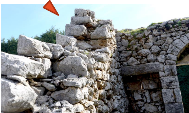
Fig. 10. My pictures showing: the ' Kalline ' walls; double-stone rows, cut from the outside and uncut from the inside
