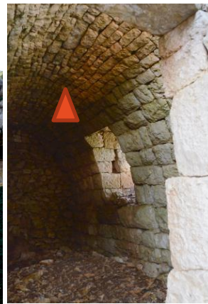
Fig. 11. Vaulted ' Abou ' with curved window with a row of small key stones
