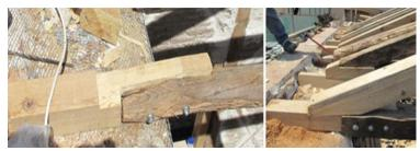
Figure 9. Prosthesis application with steel screws [30]
