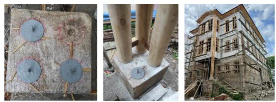
*Figure 5.* Complete replacement on the historical wooden stud; from left to right: fixing metal plates to the rock, fixing new wooden studs to the metal plate, view of wooden studs from the frontal facade [23].
