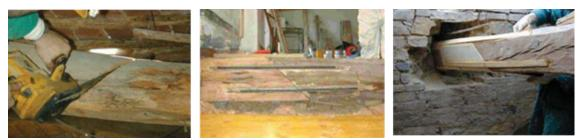
*Figure 12.* The beam end prosthesisation effort made with FRP rods are performed in the following order: inclined cut of decayed end, linking grooves and insertion of a final wedge [31]
