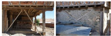
Figure 6. (a) Use of support struts in house number 7 (b) Use of diagonal braces in house number 69
