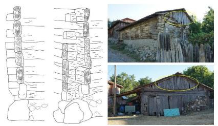
*Figure 4.* The joint detail of the kurtboğaz technique and the covering of the front wall with vertical wooden timbers
