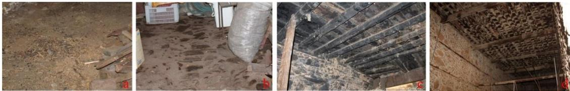
**Figure 2.** The flooring system of traditional houses in Alanya's rural region ((packed soil flooring (a), slate stone pavement (b), single timber cross-girder flooring system (c), and double timber cross-girder flooring system (d))
