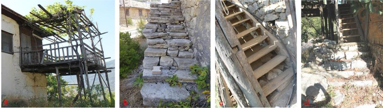
**Figure 3.** Example of cantilever (a) and types of stair (stone stair (b), wooden stair (c), mixed material stair (d)) of traditional houses in Alanya's rural region
